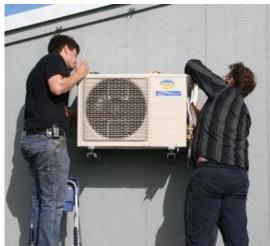
What is a heat pump and how does it work? Heat pump works the same way as a refrigerator. Refrigerator moves heat from inside the refrigerator out for him and deliver him into the cold frame (heat exchanger) back on. Heat pump heat loads in some sort of heat source and give it back in the reactor system in the house at a higher temperature.
